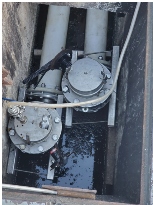
Figure 4: Initial inspection of the 316 stainless steel trough and pipe. Courtesy of Bulk Solutions
