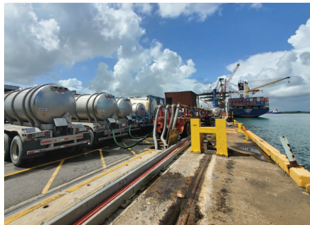
Figure 3: Connection from the pipeline to the truck manifold. © Courtesy of TOTE
