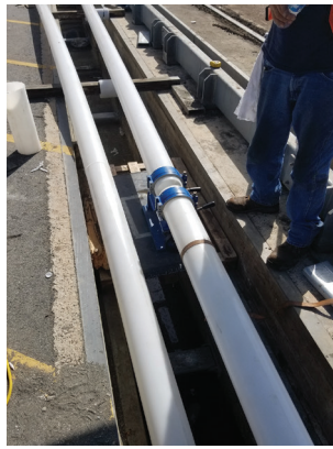
↑ Figure 7: Kynar PVDF pipe installation. 📷 Courtesy of TOTE
