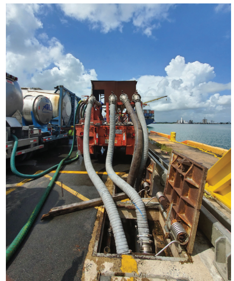
Figure 3: Connection from the pipeline to the truck manifold. © Courtesy of TOTE
